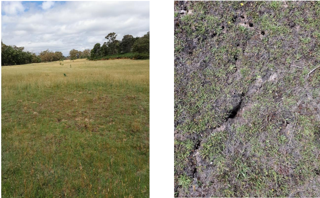
Figure 2 – Photo's showing the site of cracking clay, a mix of grey and quartzite clay, not dark heavy cracking clays expected if the site was Victorian Volcanic Plains.
