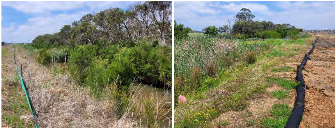
Photo 2. Photos of sediment fencing and sediment log outside the swales, in the project site.
