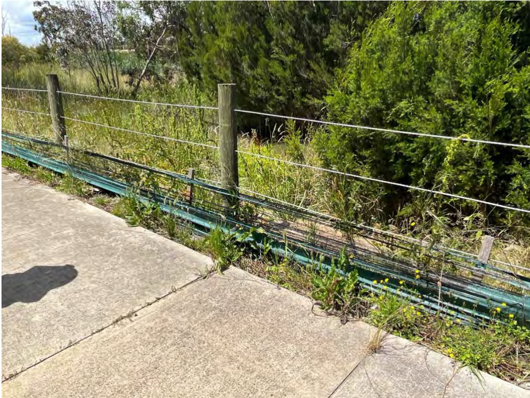
Sediment fencing along the path south of Billy Buttons Drive was generally intact but portions of it had begun to break down. The broken-down fencing must be rectified as soon as possible.
