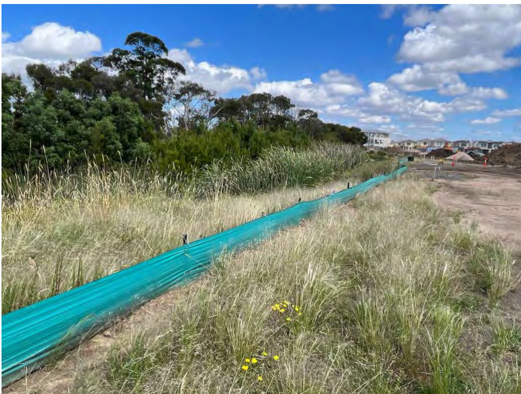
Example of sediment fencing in good condition along the northern edge of the swale in the eastern part of the study area.
