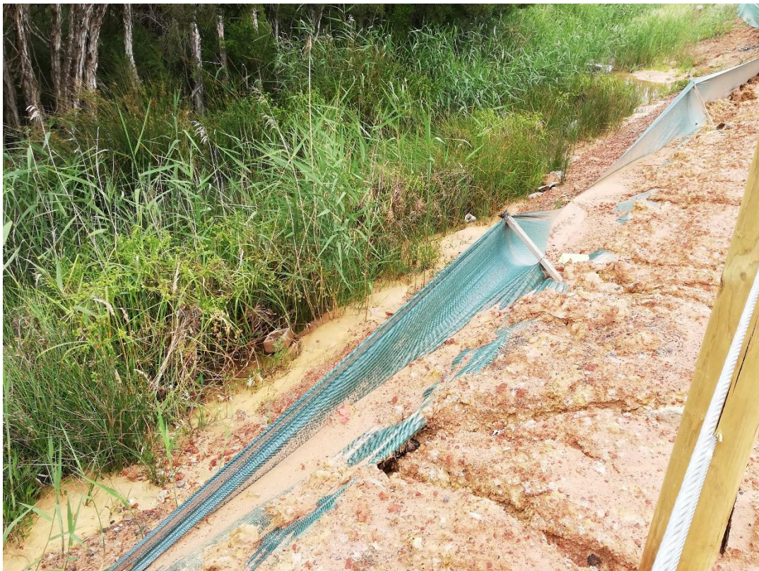
Sediment fencing has collapsed, with erosion channels running beneath the fencing, along the northern edge of the swale in the west of the site. Sedimentation of the water can be seen.
