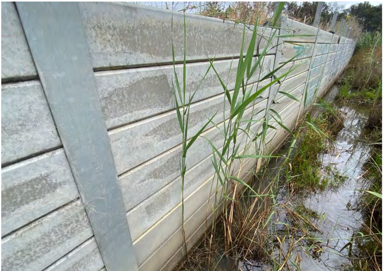
Photo 7 More open habitat at the concrete retaining wall.
