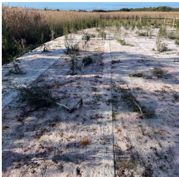
Photos 5-8. Revegetation works at refuge pools and revegetation track. Some damaged erosion matting.
