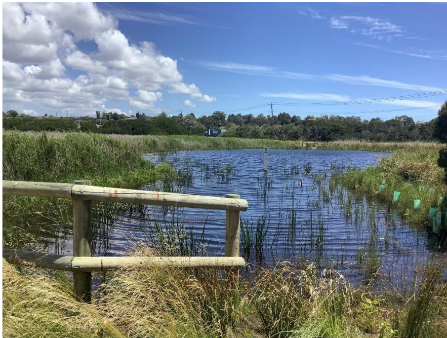
Photo 16. Tree guards surrounding the southern dam to the right of the photo
